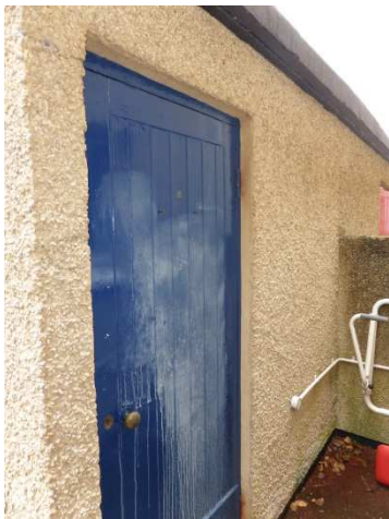
Shed doors will be repaired and painted as required
