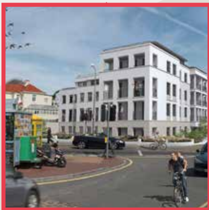
La Collette Low-Rise, St Helier 147 New Homes Due for Completion: 2023
