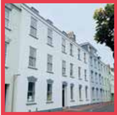
33 Belmont Rd, St Helier 3 New Homes Completed: 2021
